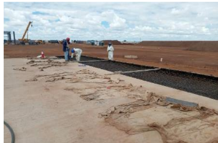
Slab Concrete Casting ongoing @ Coating Yard
