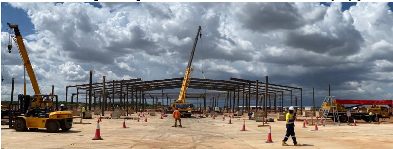
Steel Structures Erection ongoing @ Coating Yard
