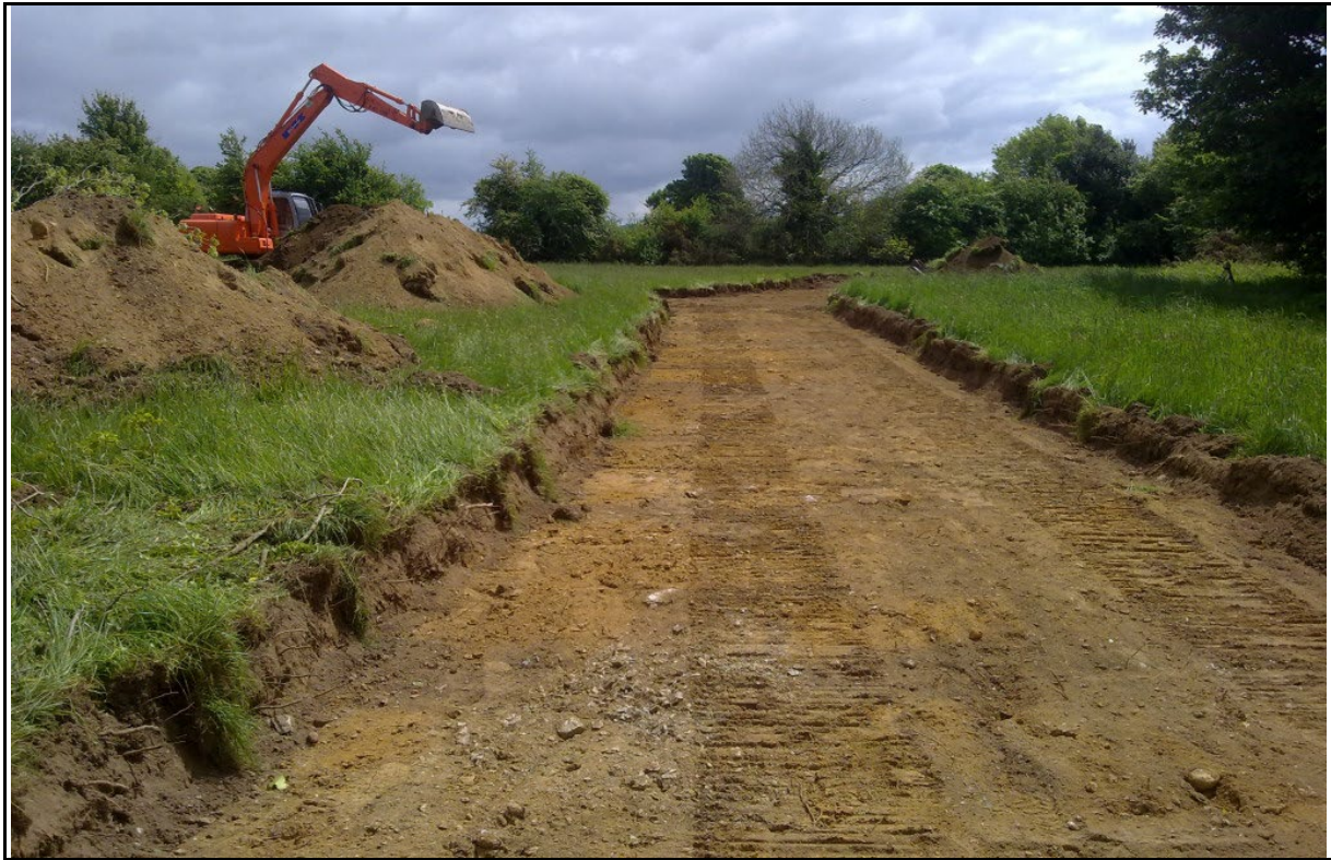
Figure 2.4-3 Typical Topsoil Removal
