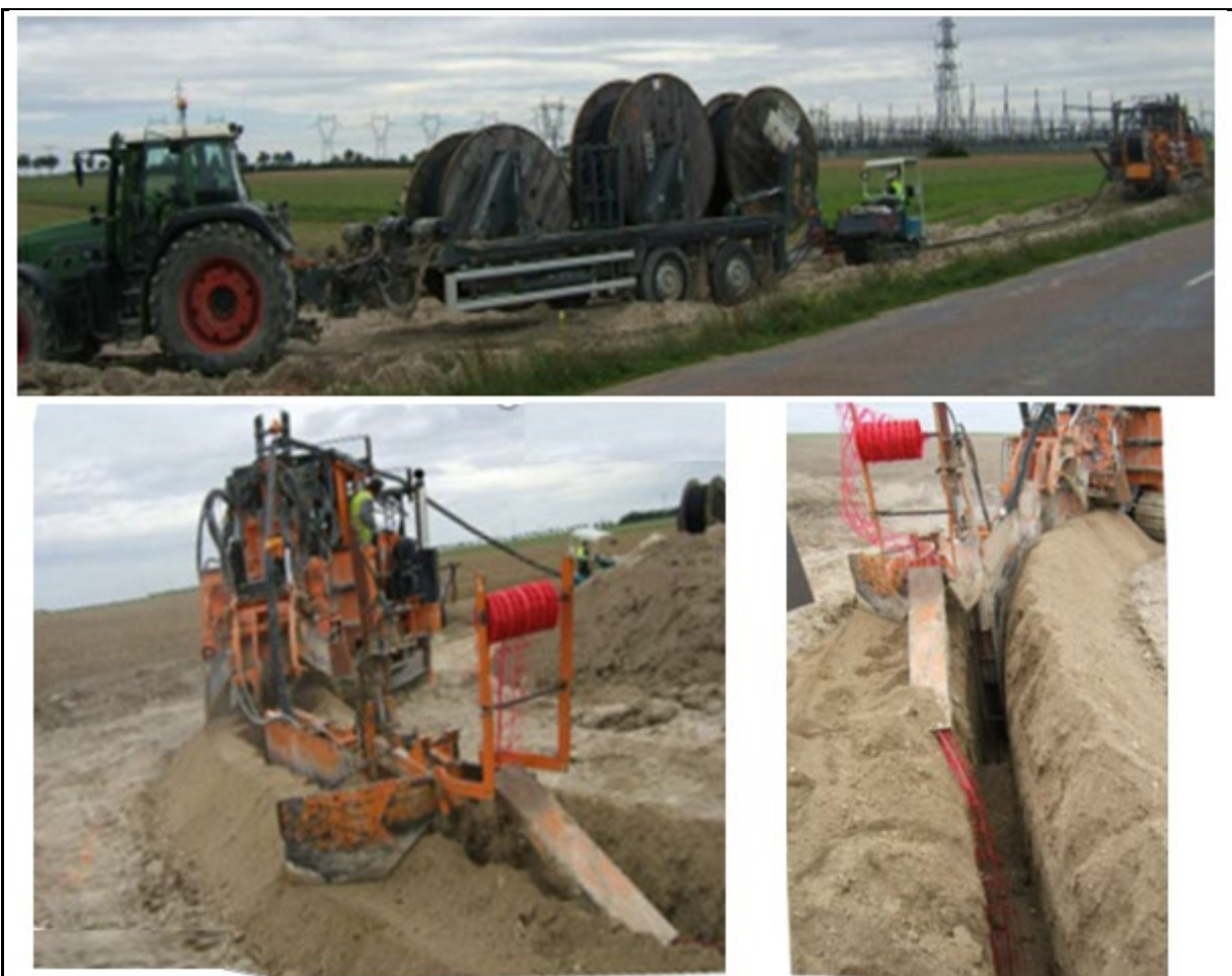
Figure 2.4-11 High-Voltage Power Cable Installation
