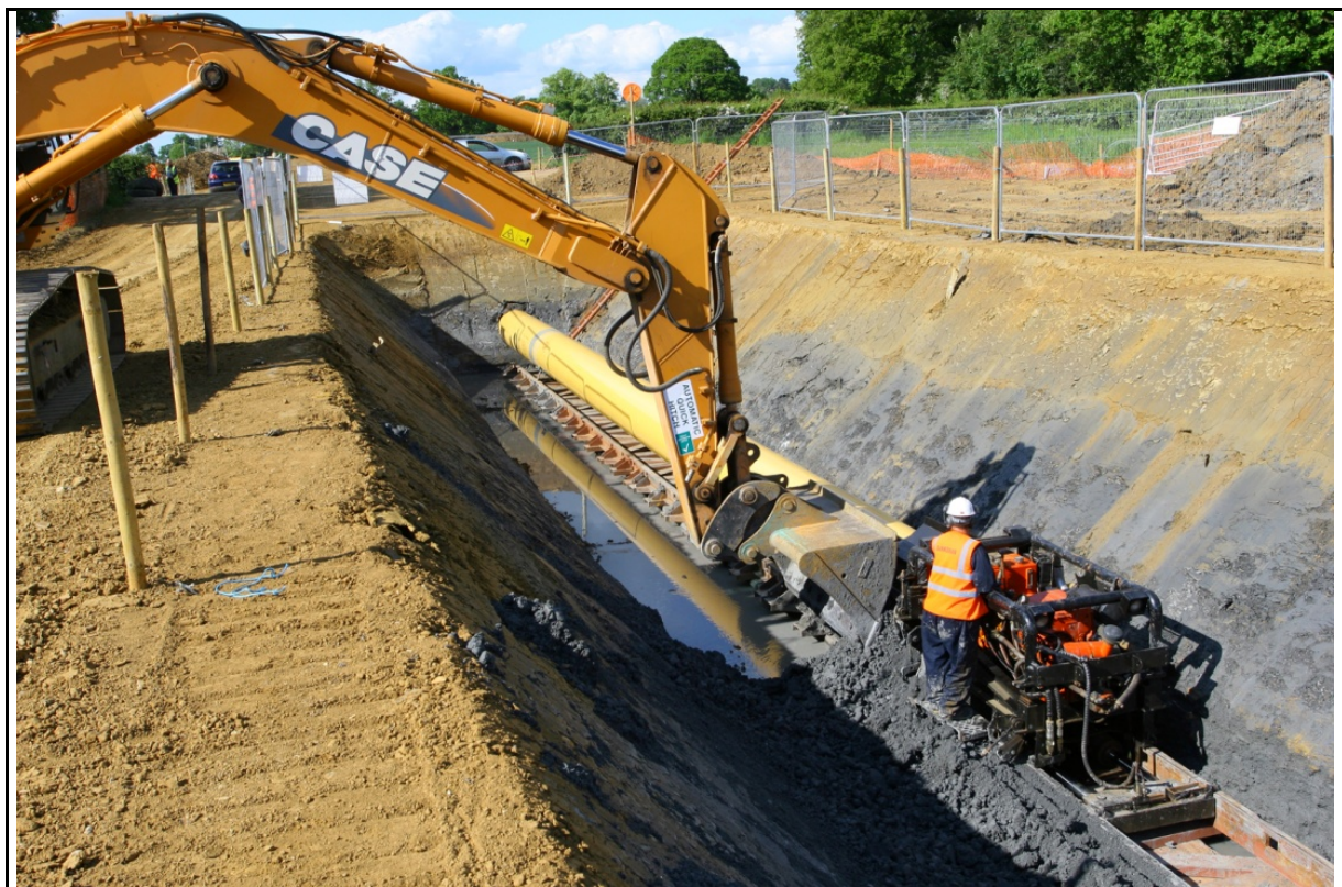
Figure 2.4-16 Auger Bore
