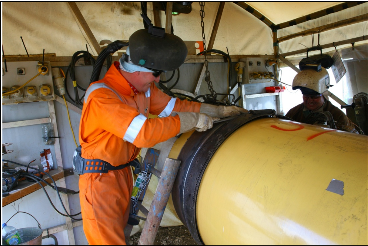
Figure 2.4-6 Typical Pipeline Welding
