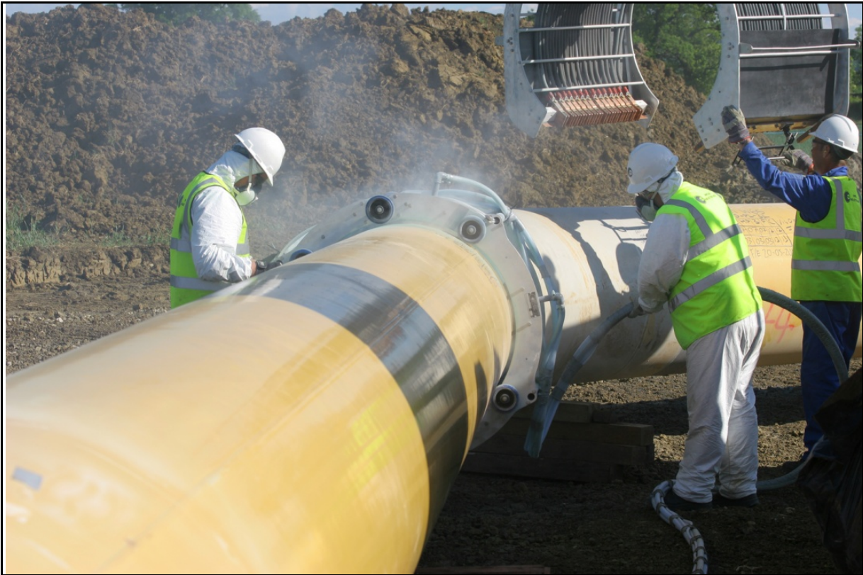
Figure 2.4-8 Anti-Corrosion Field Joint Coating
